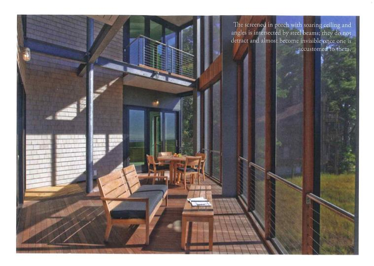
While the floor to ceiling windows and doors offer a dramatic backdrop of the marsh in every room, they still need to be structurally stable and able to withstand coastal winds. To achieve that goal, McInturff incorporated metal crossbars or tension ties that expand across some of the larger windows. They serve as braces between the steel columns, eliminating any motion during high winds or settlement while adding to the home's nautical character.
